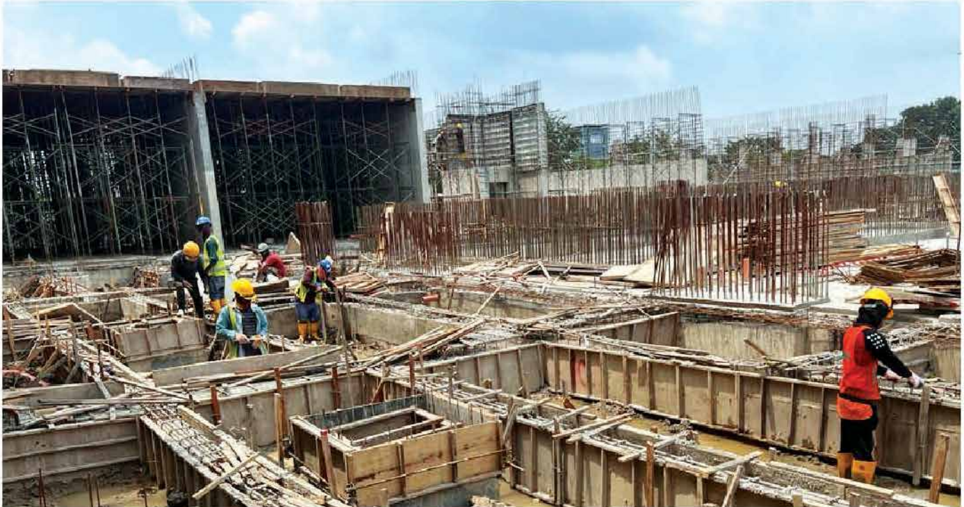
P173 A 30 storey service apartment at Gravit8 Klang [PH2C]
