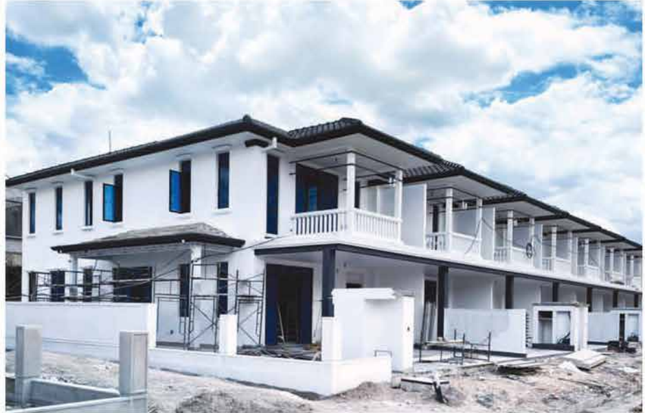
P162 176 units of gated & guarded double storey terrace houses at Eco Majestic, Semenyih
