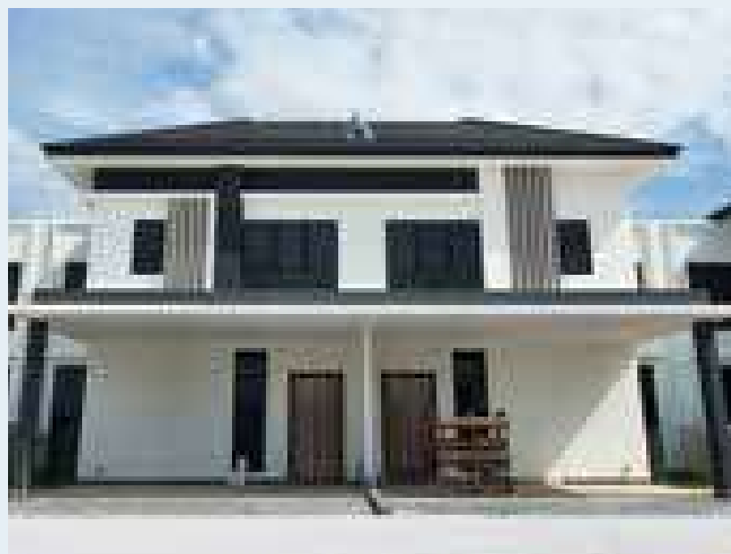
P167 104 Units gated & guarded Double Storey Terrace at Eco Ardence, Setia Alam
