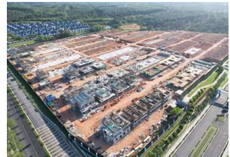
P203 - 68 units semi-detached at Cyberjaya, Selangor
