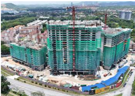
P195 - 3 blocks of apartments (450 units) at Ara Damansara, Selangor
