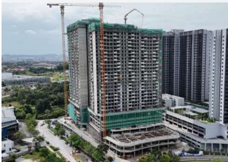
P192 - 2 blocks of serviced apartments (468 units) at Tropicana Metropark, Subang Jaya
