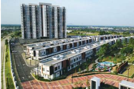
P183 - 107 units Co-Home and 1 block of 21-storey apartments (294 units) at Eco Sanctuary, Kuala Langat
